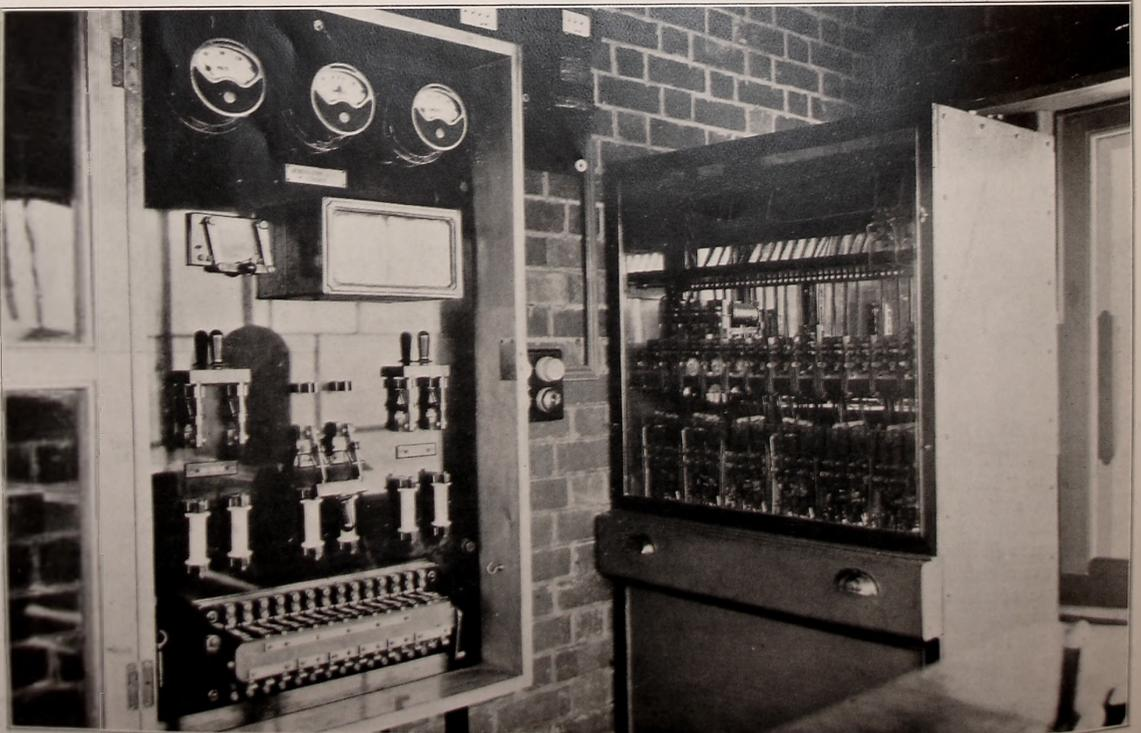
Fig. 4.—Power Switchboard (left) and Contactor Case (right) in upper part of Signal-Box. Batteries in lower part of Signal-Box.
