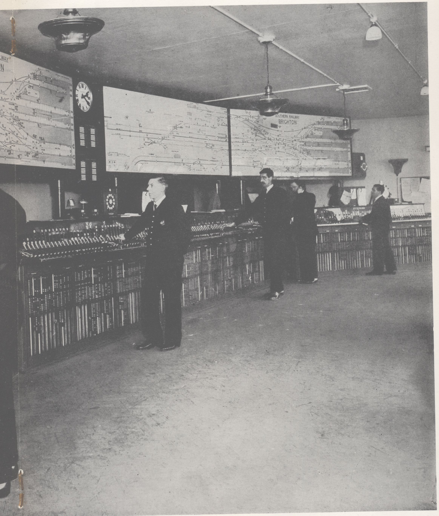
bin with 225-lever all-electric Interlocking Frame.
