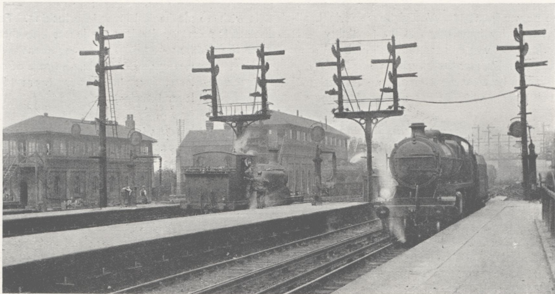
Brighton Station Starting Signals, etc. Before alteration.
