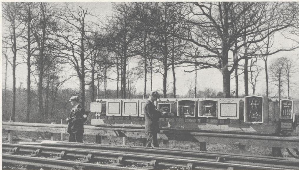
Automatic Signal location, Apparatus Cases with Relays, Track Feed Sets, etc.
