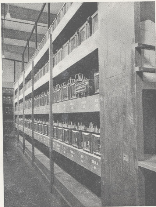
Relay Room, Brighton.
