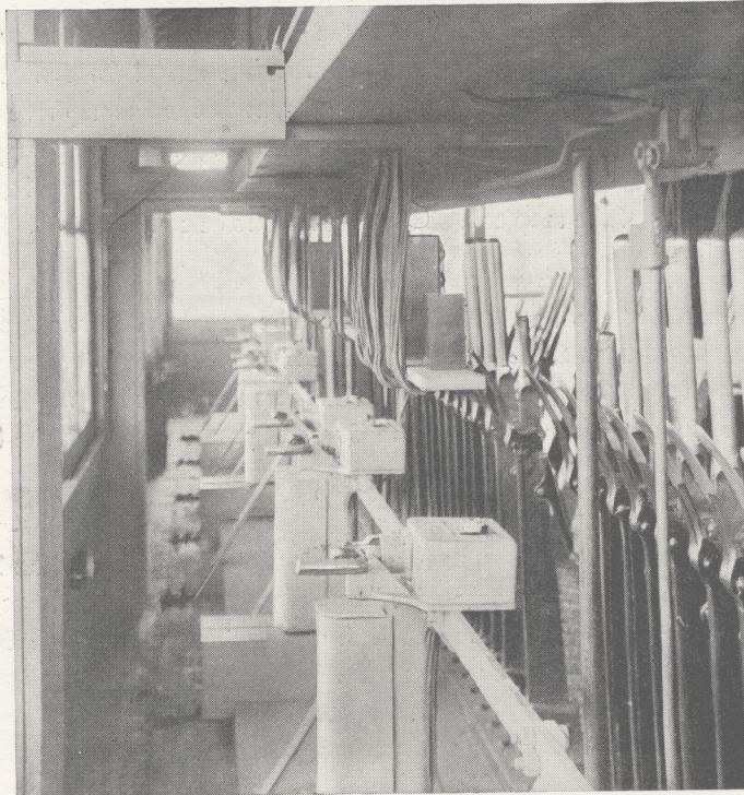
Point Machine Crank Handles and interlocked Circuit Controllers—Earlswood Junction Cabin.
