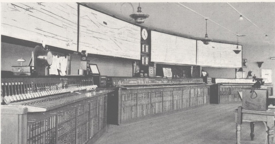
Interior of the new Cabin showing 225-Lever Power Frame with all-electric interlocking.
