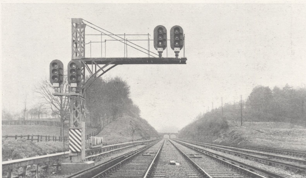
Up Home Signals, Copyhold Junction.
