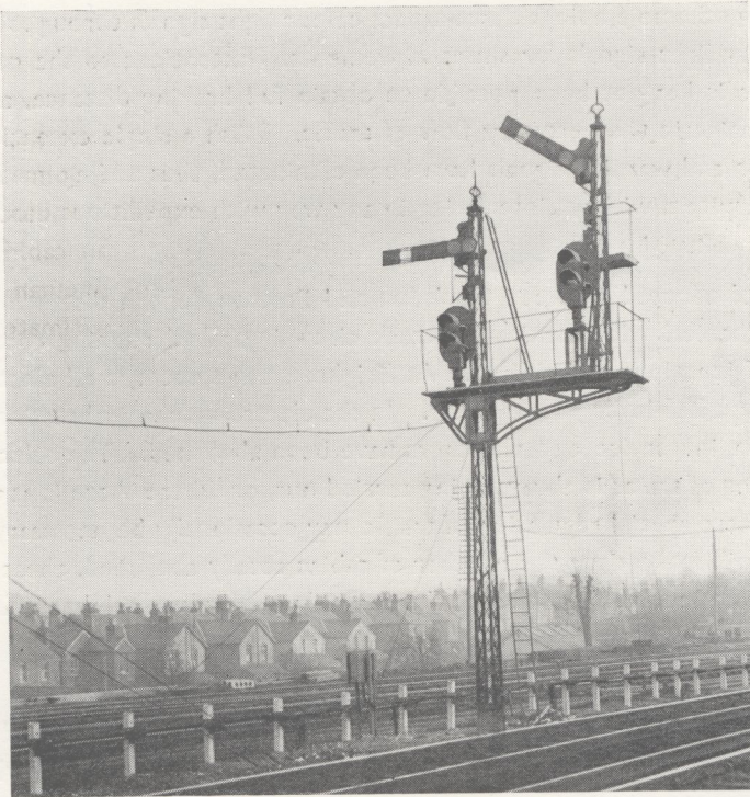
Upper-quadrant Semaphore Signals, with 2-aspect Colour-light Distant Signals—Earlswood Junction.
