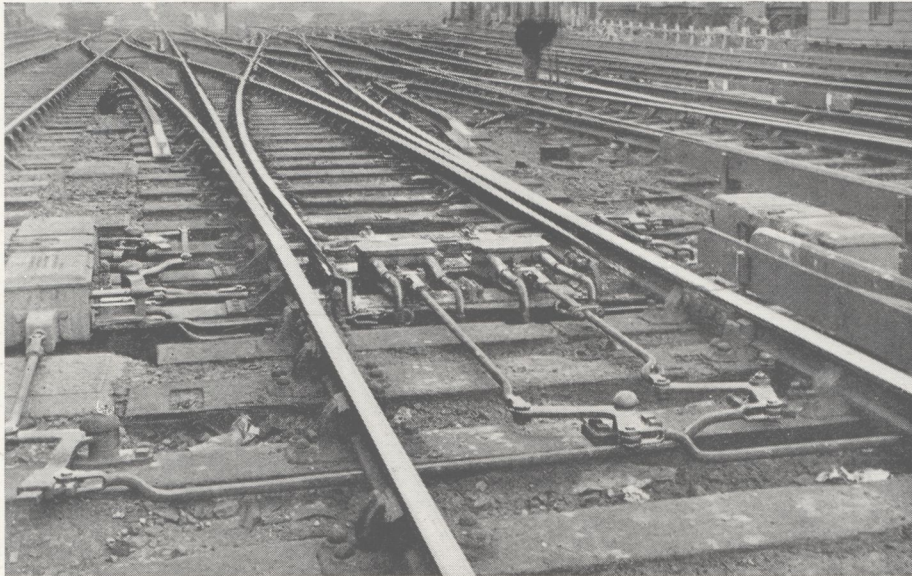
Three-throw Point Layout operated by two Style M3 Point Machines.
