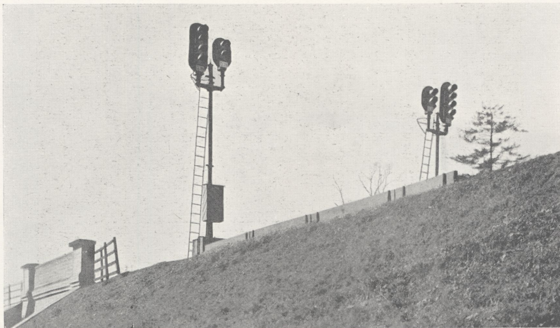
Two signal masts on the embankment at the station, each with two signal heads.
