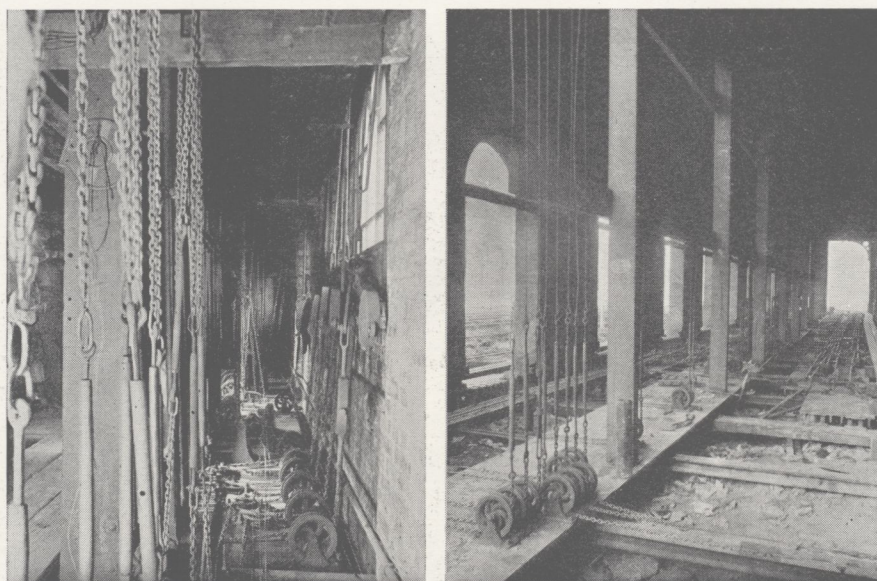
Mechanical Point and Signal Connections under old cabins at Brighton, now removed.
