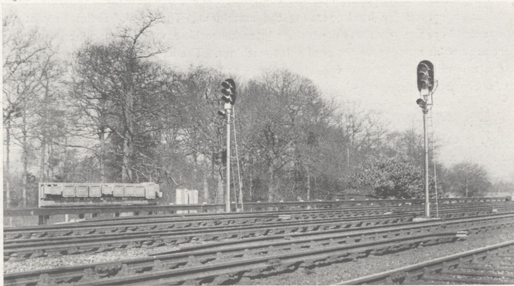
Automatic Signals between Three Bridges and Gatwick.
