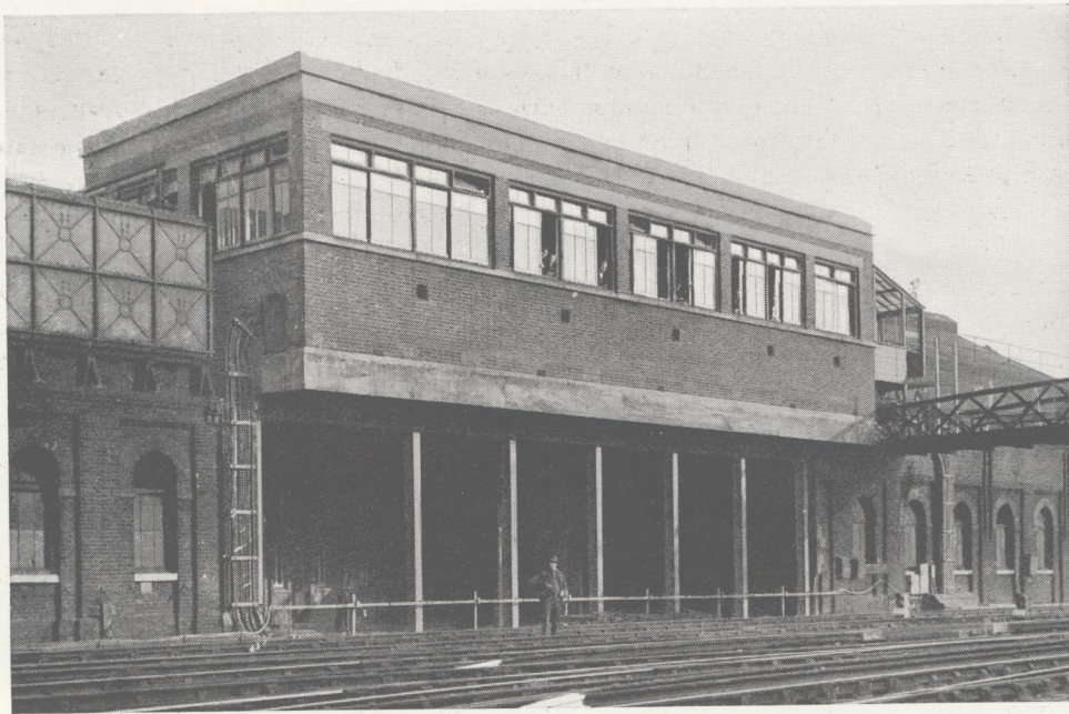
Exterior of new Signal Cabin, Brighton.
