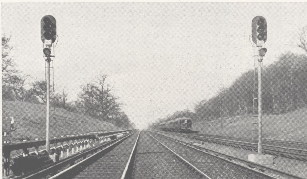
Automatic Signals, Up Line between Three Bridges and Balcombe Tunnel.
