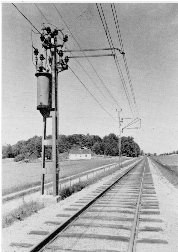
Fig. 8. For the Malmö lines and for the further electrifications the booster transformers are put on the poles as shown in this figure.
