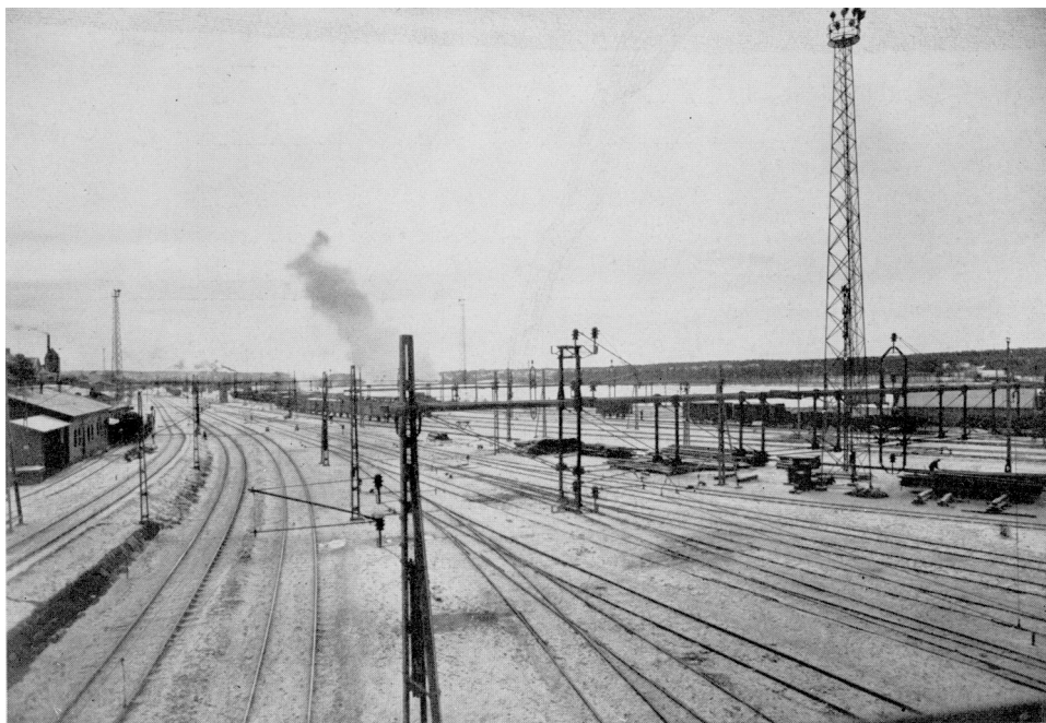
Arrangements and steel towers for the lighting of yards. Day-time.
