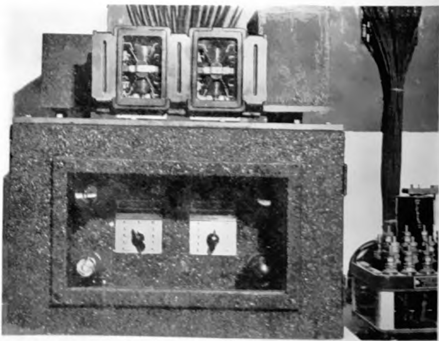
One unit of the carrier apparatus at Las Vegas
