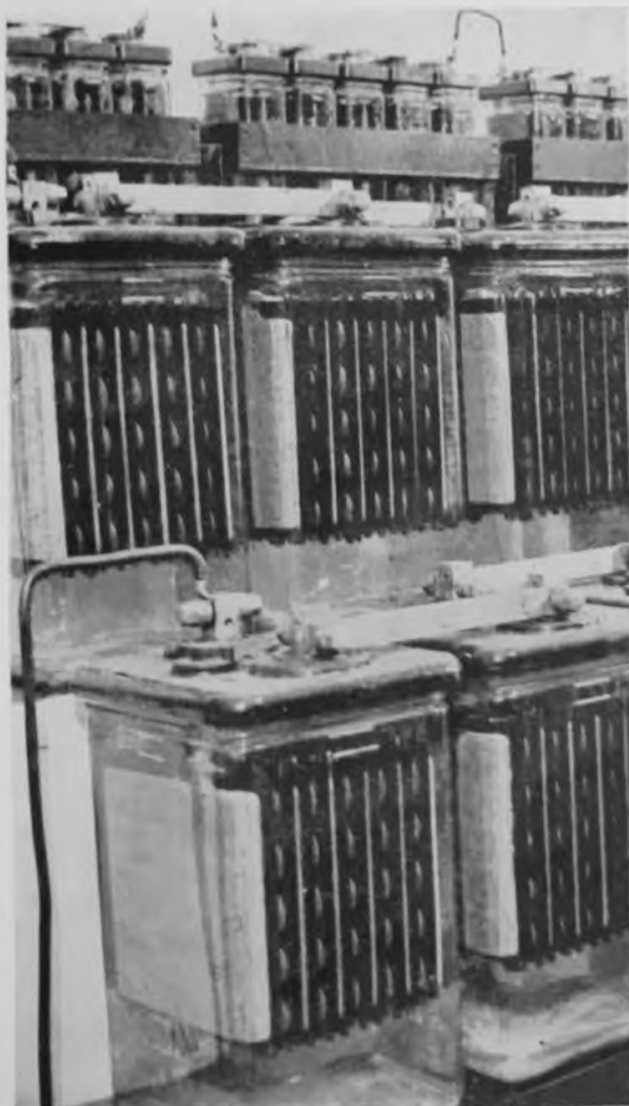
Storage battery for feeding the C.T.C. coded line circuits, local code equipment, and the various relays that are located in the Las Vegas office
