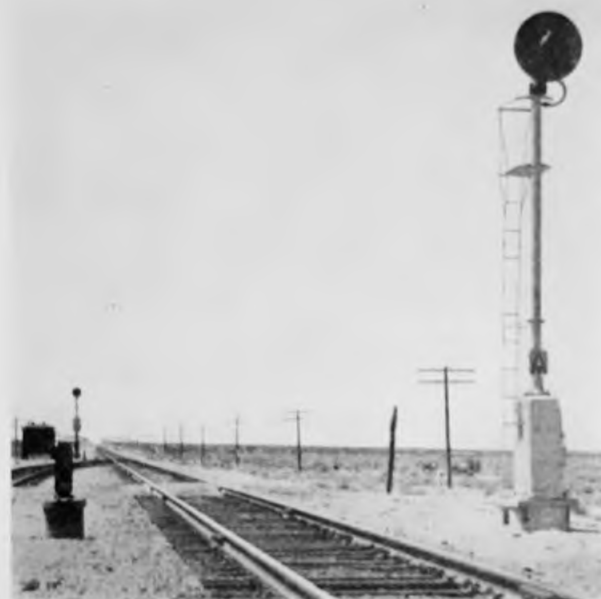
Dwarf and high signals at the west end of the Roach siding at which there is a handthrow switch and electric lock
