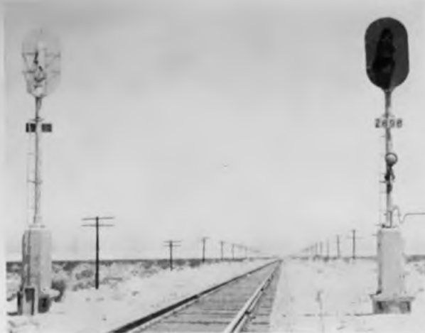
The automatic signal in approach to west end of Roach, note operative lamp on mast. Below—Signal at west end of the siding at Roach with "S" lamp in the lower unit to indicate the electric switch lock is unlocked
