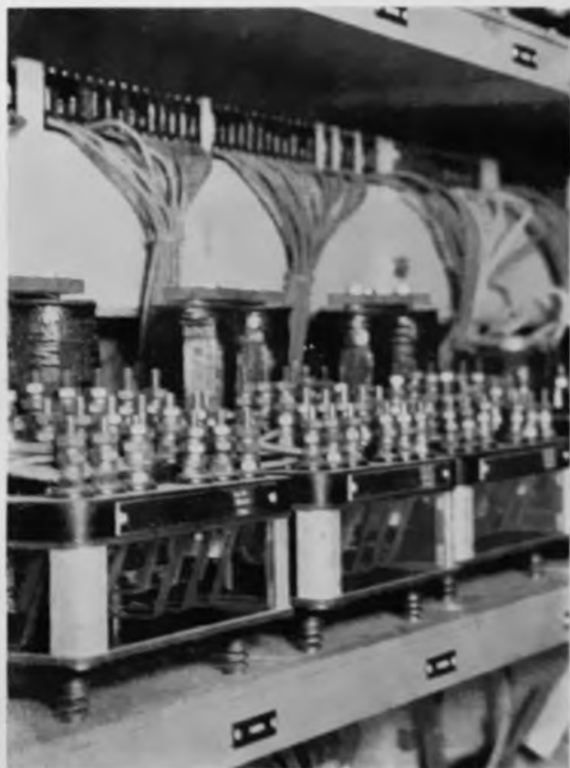
The wires from relay terminals each go through a separate hole in the back panel with the tag around the wire tacked to board
