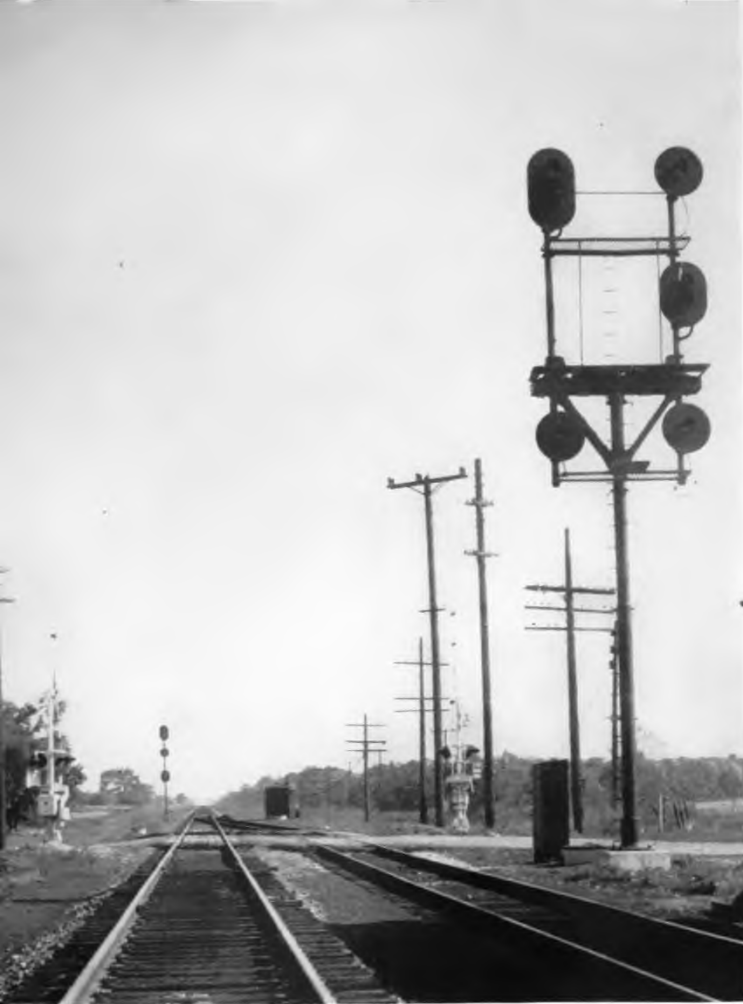
Main track station-leaving signal and leave-siding signal are on one bracket mast
