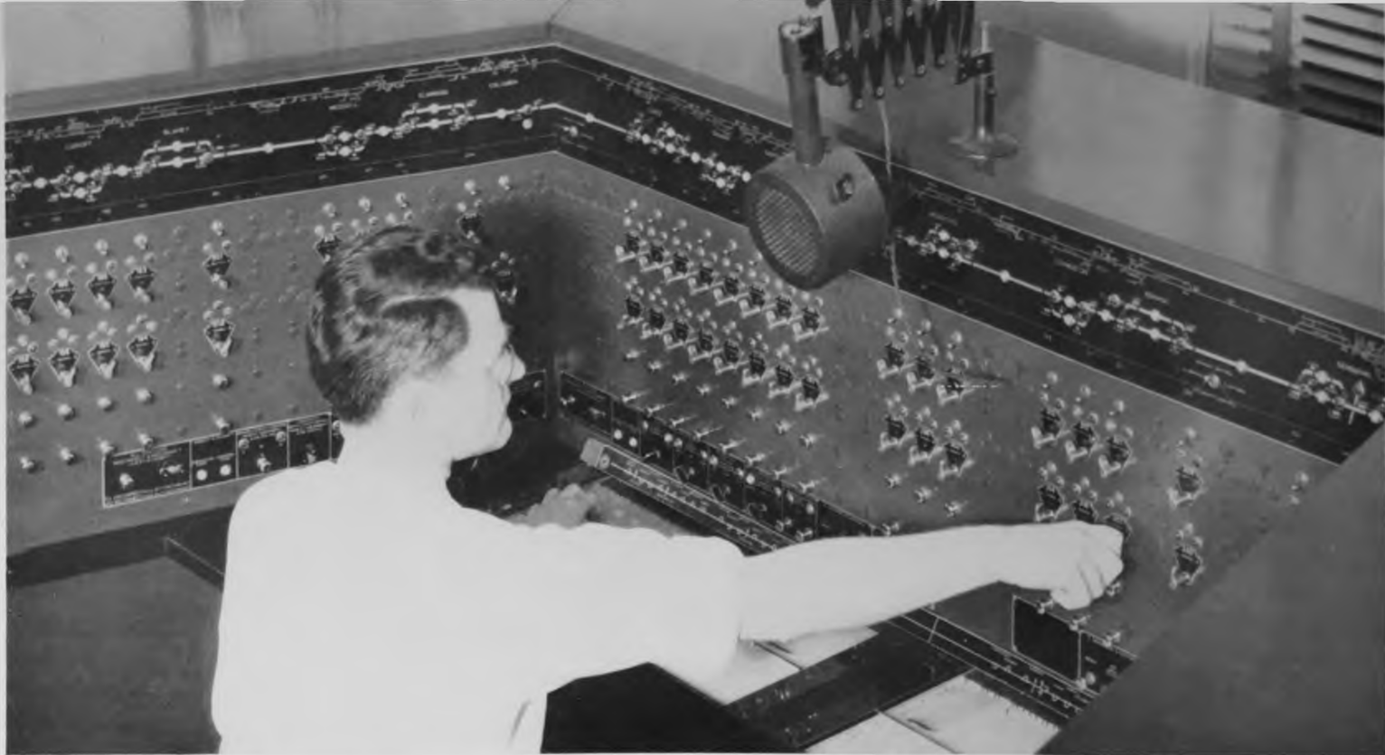
This machine in the dispatcher's office at Savannah controls the entire 248 mi. between Savannah and Hamlet
