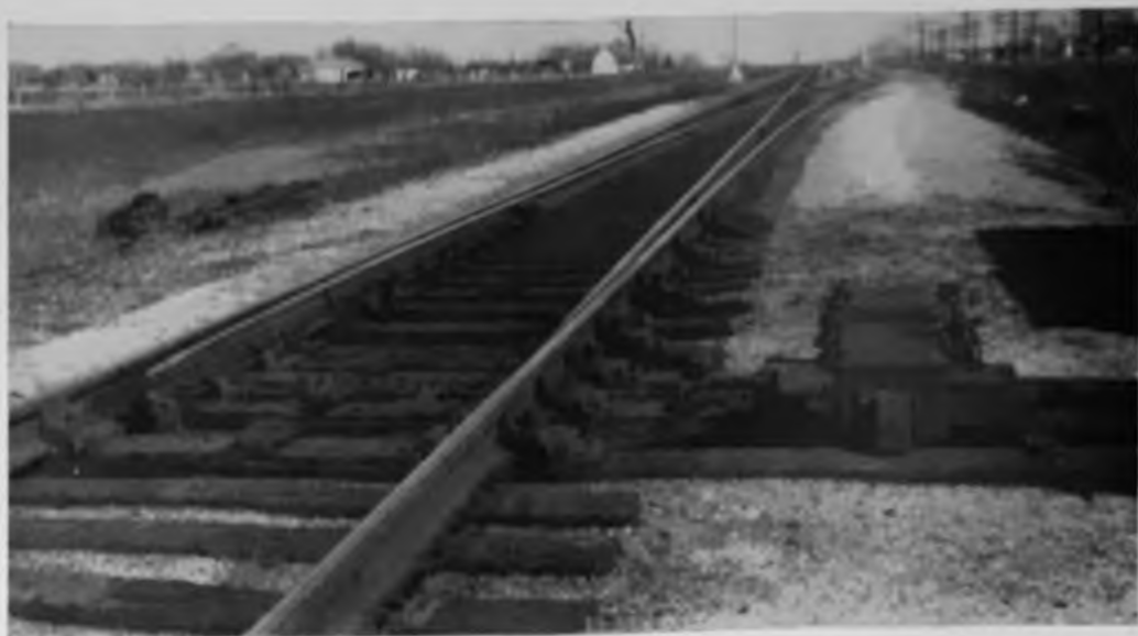
New No. 15 turnouts, permitting train speeds up to 25 m.p.h., were installed at the power-operated sidings
