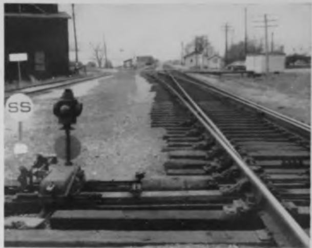
Trains normally depart from the end of the siding which is equipped with a spring switch
