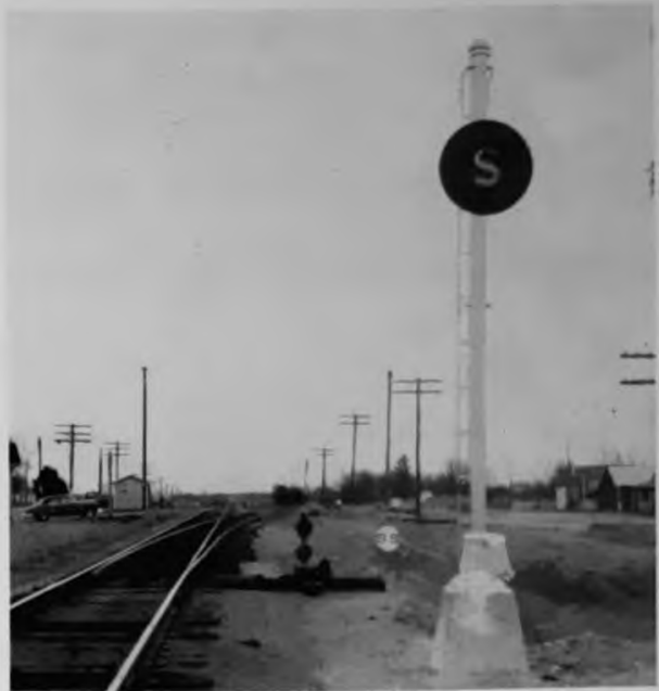
If a train, approaching on the main track, is to be directed to enter a siding at the spring switch end, the indicator shown here is controlled to display the letter "S"
