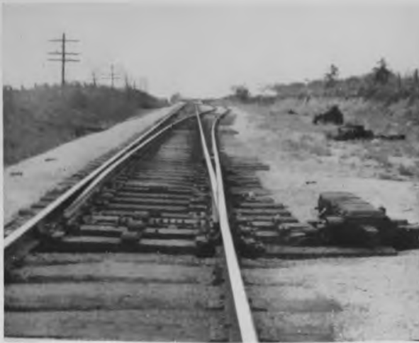
Trains normally enter a siding at the end with dispatcher-controlled power switch and signals
