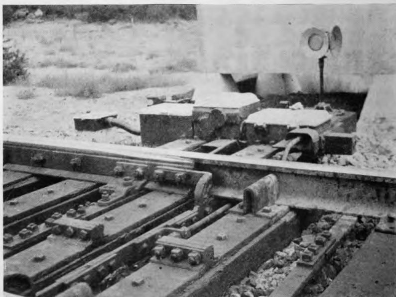
The power switches have heavy gage plates and adjustable rail braces on four ties
