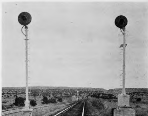
The west end of a siding showing a high leave-siding signal at the left
