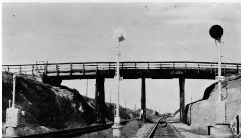
Automatic signals on the siding located just west of Mountainair station
